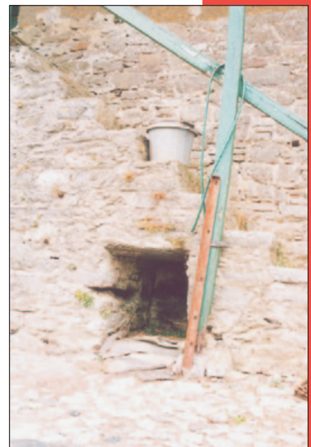
Right: Not unique, but certainly rare, these stone steps giving access to a granary have a dog kennel built-in..... across the yard from the farmhouse door.
