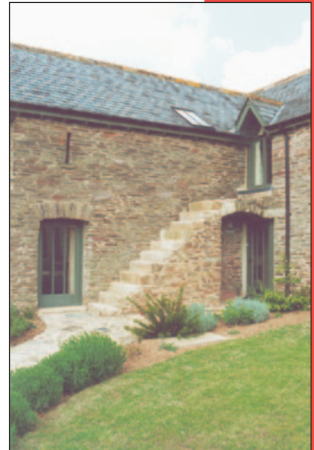
Right: Although conversion made these characterful steps redundant they were nevertheless retained as a feature of interest and a reminder of how the building was formerly used.
